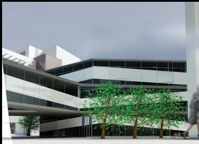
Steel, glass and concrete provide the three-story design structure. Photochromic exterior glazing strips adjust according to the amount of daylight.
